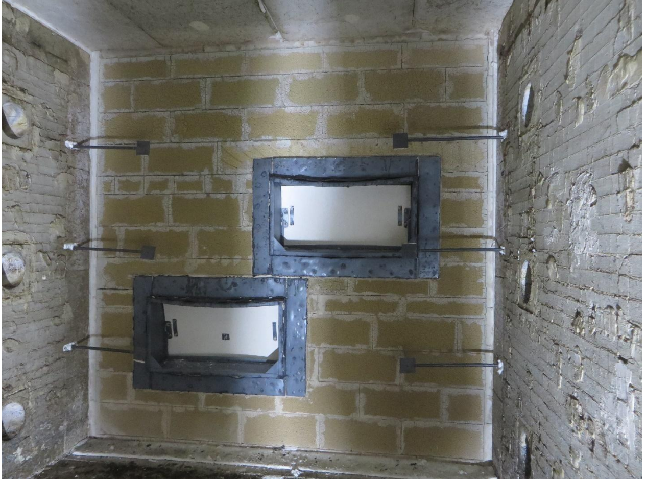
Photo C4: Exposed side after the fire test
